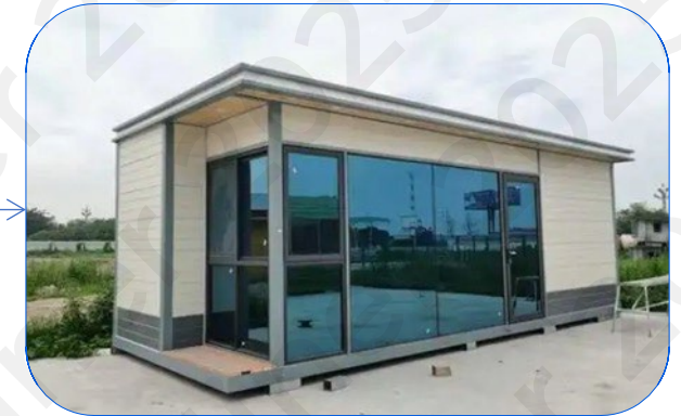
• Operations and Maintenance Office Container
